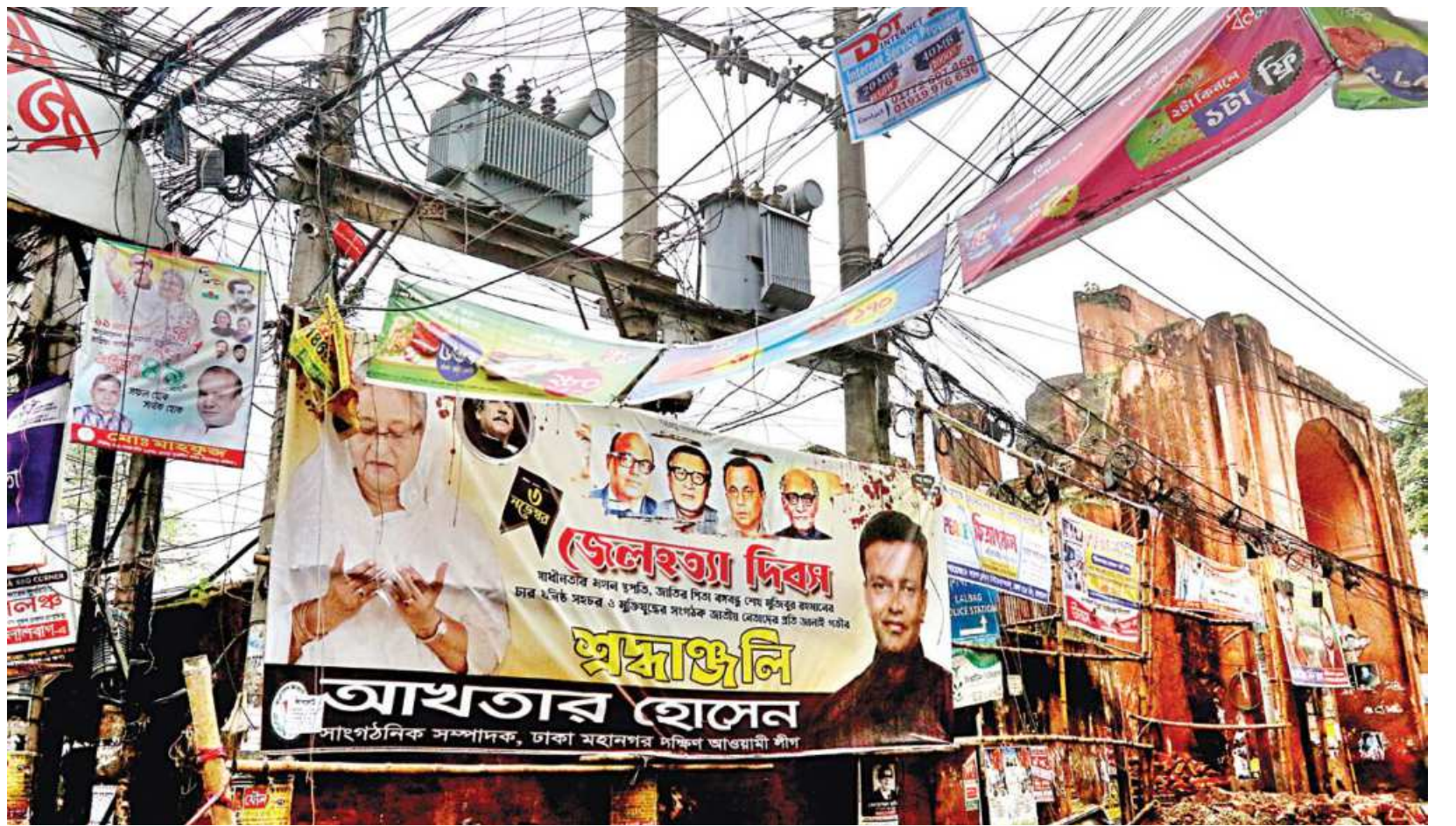
Banners hanging from electricity poles and tangled webs of cables mar the beauty of the entrance to Lalbagh Fort, an architectural jewel of the Mughal Empire, in Old Dhaka. The photo was taken yesterday.
