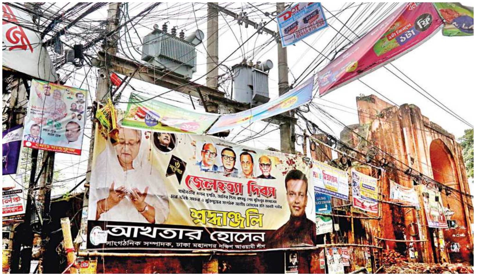
Banners hanging from electricity poles and tangled webs of cables mar the beauty of the entrance to Lalbagh Fort, an architectural jewel of the Mughal Empire, in Old Dhaka. The photo was taken yesterday.
