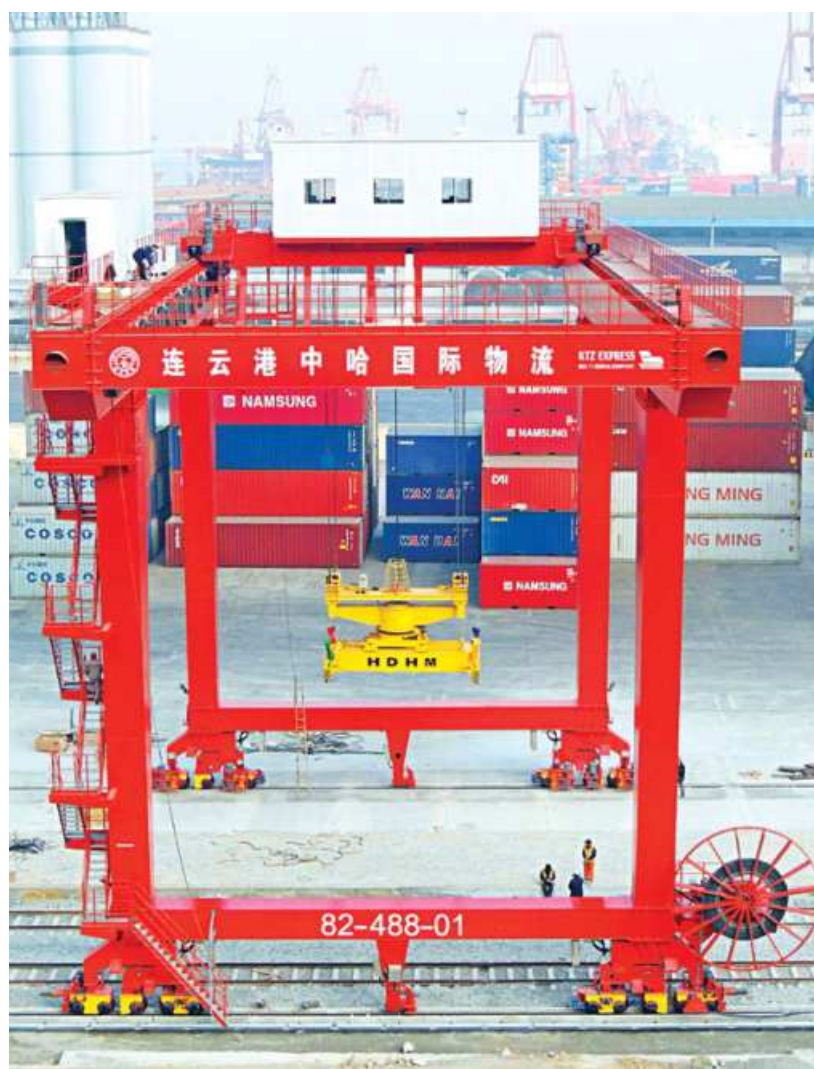
Chinese workers checking on the giant container crane at the port in Lianyungang, China's Jiangsu province.
