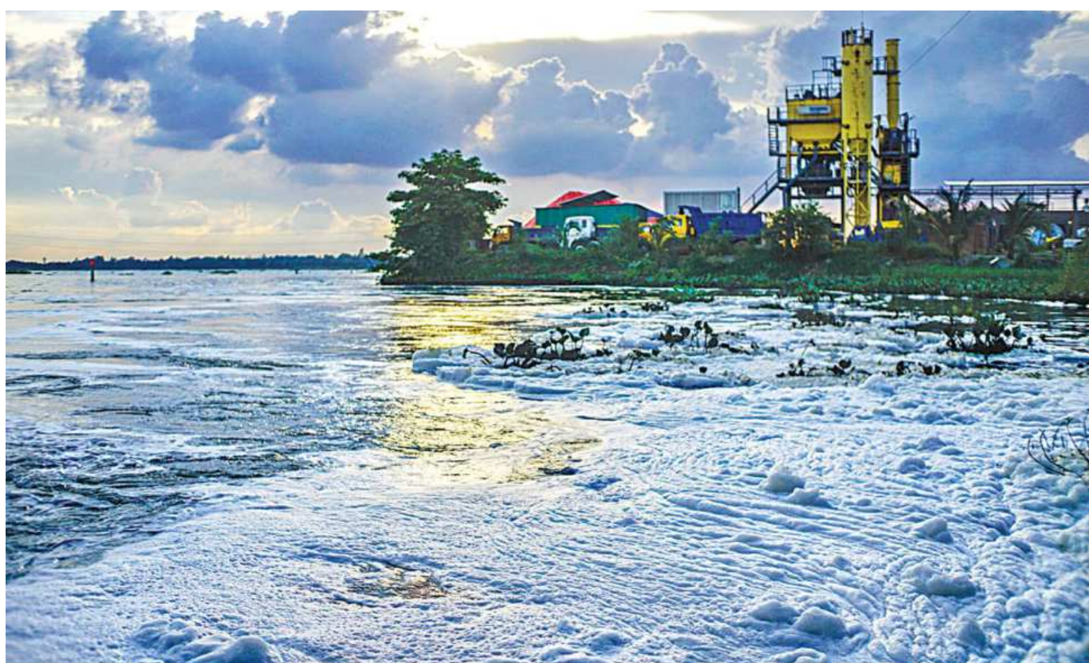
When accumulated water from low-lying areas of the capital overflows, a pump of Water Development Board at Goranchatbari is turned on, draining all of it into the river. The only problem is this water comes from residential drains and factories, which means it is contaminated to a horrifying degree, and hence the foams by the shore. This photo was taken recently from Mirpur-Ashulia-Beribadh Road. PHOTO: RASHED SHUMON
