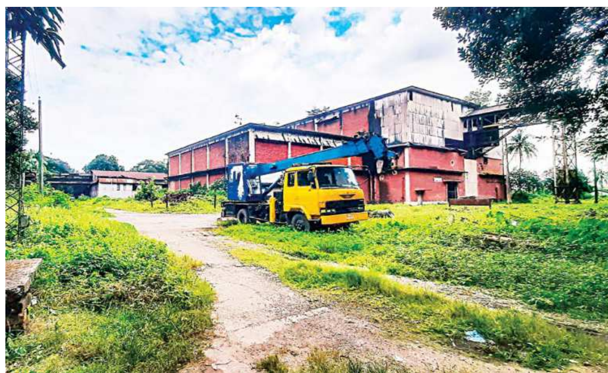
Production was stopped at Khulna Newsprint Mills about 20 years ago for continued losses and capital shortages. Amid overgrown weeds and bushes all around, now it looks like a ghost town, with machinery rusting away and buildings losing strength. The photo was taken recently.
