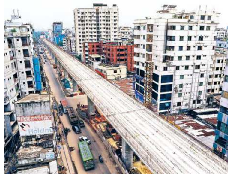
A view of the Dhaka Metro Rail project.
