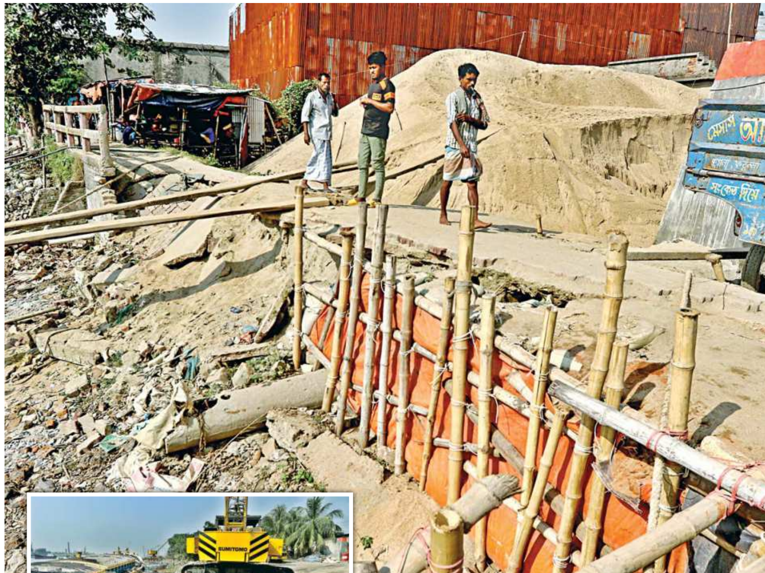
A part of the walkway along the Buriganga collapsed in Narayanganj's Munshikhola. The mooring of cargo vessels in the area has been causing damages to the walkway for about a year. Inset , a crane is deployed on the shore of the river to unload goods from boats. The photos were taken yesterday.
