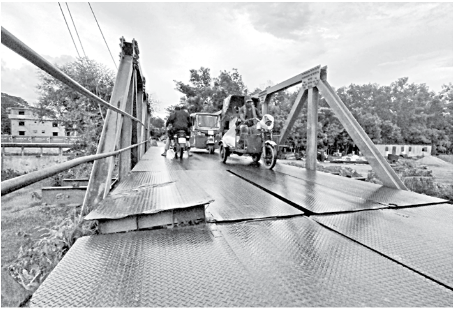
A still plate of the iron-structured bailey bridge on the Fanaí river in Moulvibazar's Kulaura upazila is seen displaced, hampering vehicular movement.
