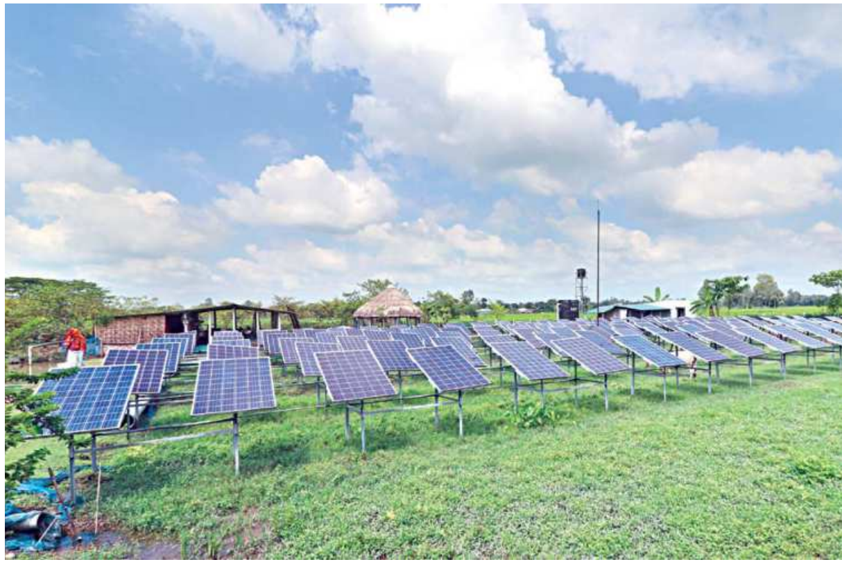
A solar irrigation facility at Nizpara village in Dinajpur's Birganj upazila. Farmers in the remote village where electricity is yet to reach get the water supply thanks to the solar-run system to irrigate their land.
