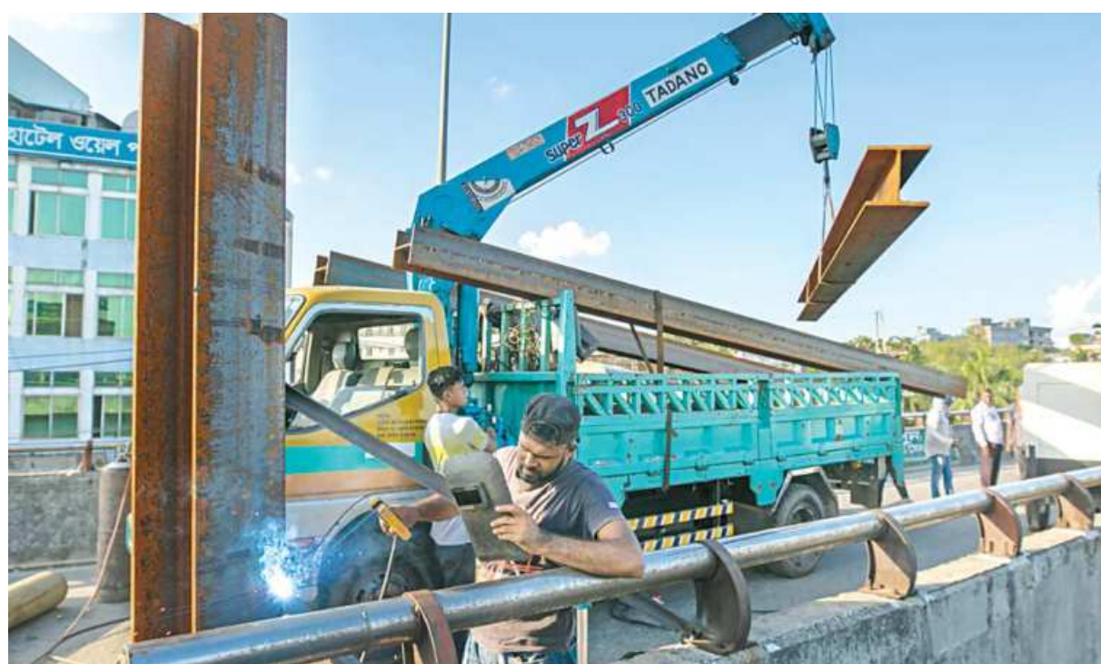
Closed due to fears over cracks emerging on its surface, the port city's MA Mannan Flyover's Kalurghat-ramp is getting height barriers installed to control movement of heavy vehicles. This photo was taken from Bahaddarhat area yesterday.
