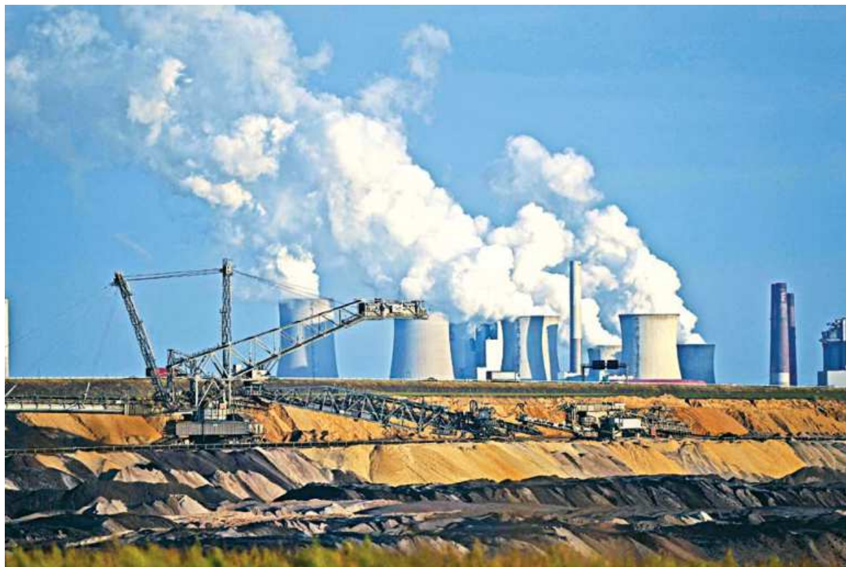
Open-cast lignite mining is seen near the coal-fired power station Neurath of German energy giant RWE in Garzweiler, western Germany on October 27.
