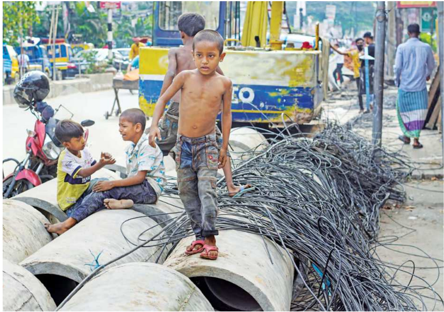
ALL FUN AND GAMES UNTIL... On the capital's CR Dutta Road, these concrete pipes have become an obstacle course for children. The little ones, however, are unaware of the risk of injuries they pose. Amid Dhaka South City Corporation's development work, the pipes have been lying there haphazardly for some time now. Besides pedestrians and vehicles being inconvenienced by this whole situation, the kids often get hurt while playing with the pipes as seen in the background. This photo was taken yesterday.
