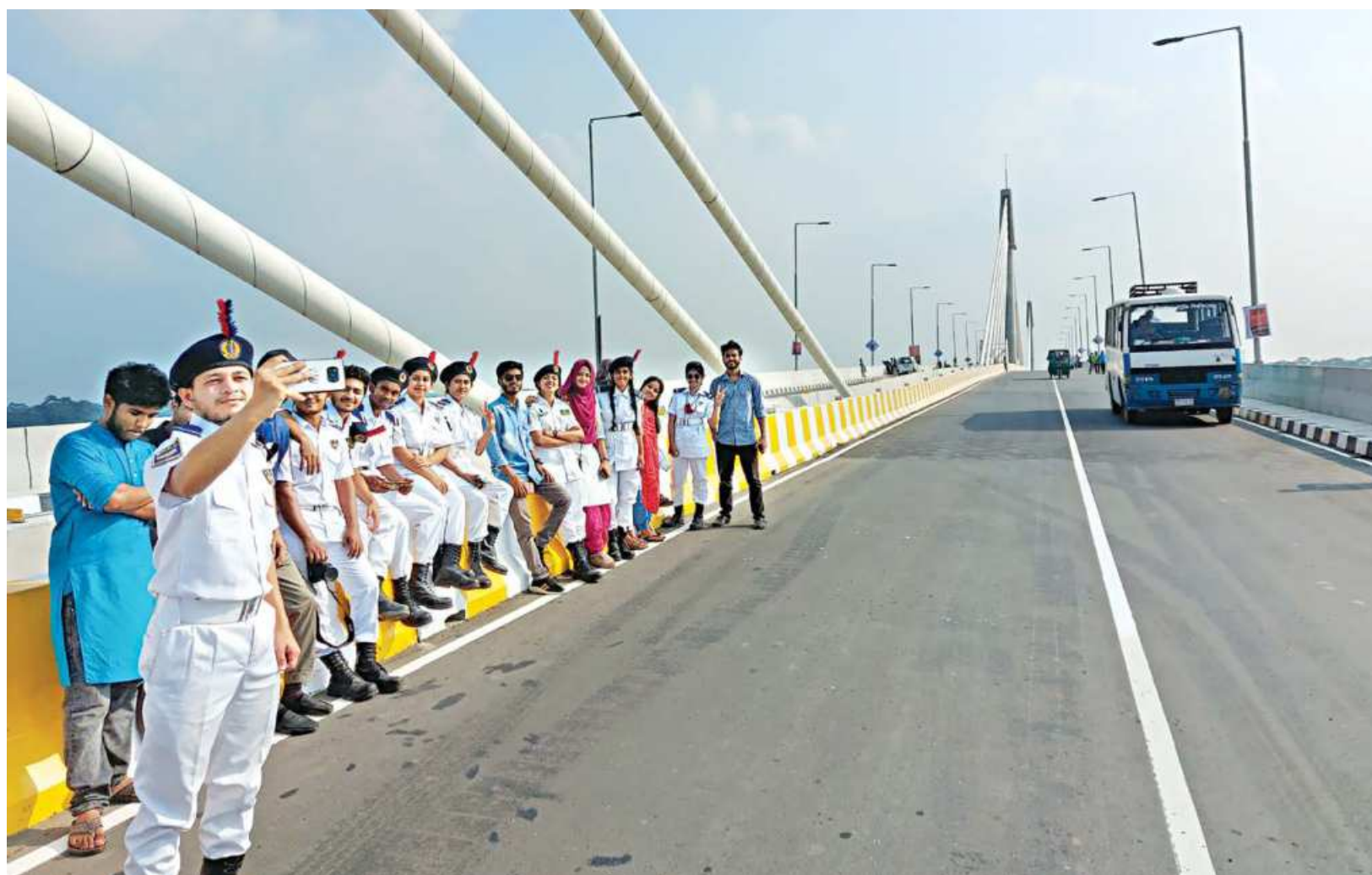
People taking photographs on the bridge constructed over the Payra river in Lebukhali on Patuakhali-Barishal highway after Prime Minister Sheikh Hasina inaugurated the four-lane bridge virtually from the Gono Bhaban yesterday.
