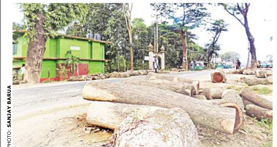
Around 1,400 of the trees were rain trees. Before being cut to facilitate construction of the 11.05-kilometre connecting road, they stood on both sides of the road stretching from Anwara upazila's Choumuhoni area to Shikalbaha of Karnaphuli upazila.
