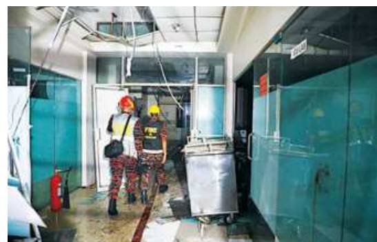
The fire originated at the ICU of the hospital yesterday noon, which left at least 10 persons injured. Seven firefighting units doused the blaze around 2:15pm.
