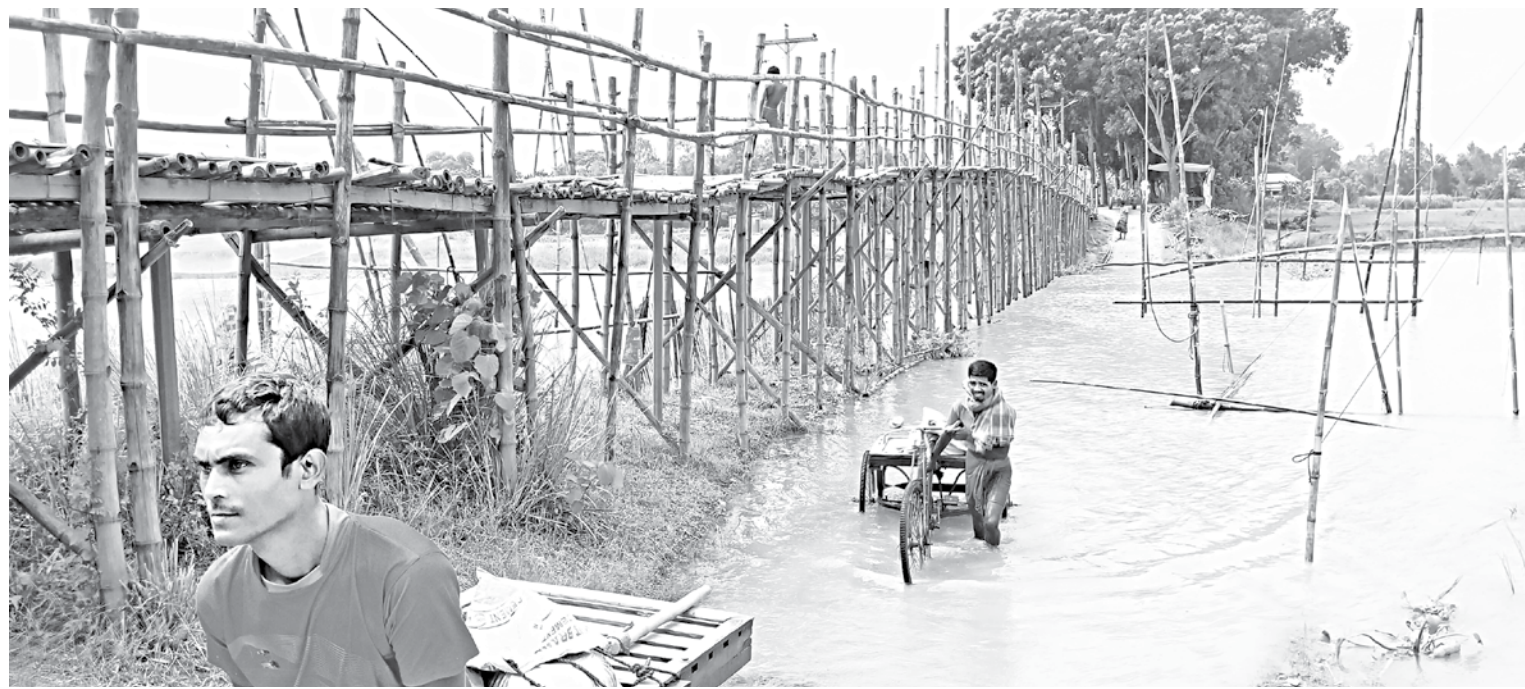
People of different villages under Mokna union in Tangail's Nagarpur upazila often have to wade through knee deep water to cross this small branch of the Dhaleshwari river as there is no permanent bridge.
