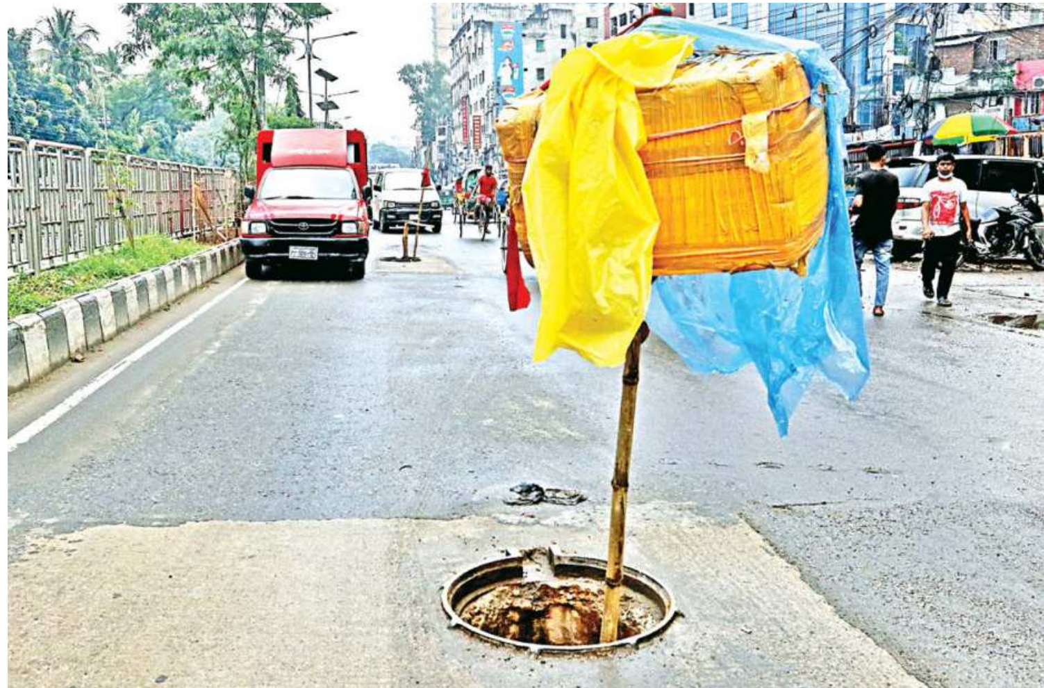
Right down the middle of this busy road at the capital's Fakirerpool, a couple of manholes are missing their covers. This is heavily disrupting vehicular movement, as they have to make their way around the holes in order to avoid accident. Finding no other way, some locals have stuck whatever they can -- sticks, bags, and even containers -- into the manholes to alert commuters of their location. This photo was taken recently.
