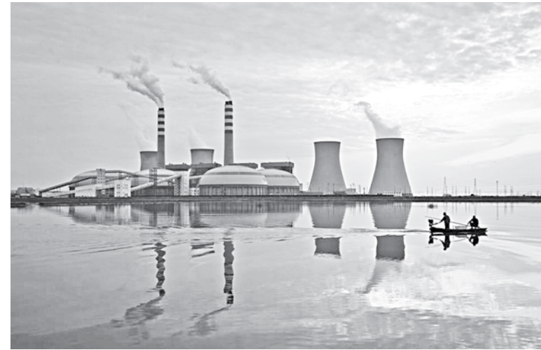
Fishermen sail a boat past a power plant of the State Development and Investment Corporation outside Tianjin, China on October 14.
