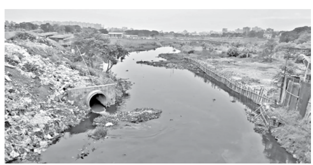
This is the pipe leading to the New Road canal that Manik came out of. He was found lying on the canal's shore some six hours later.
