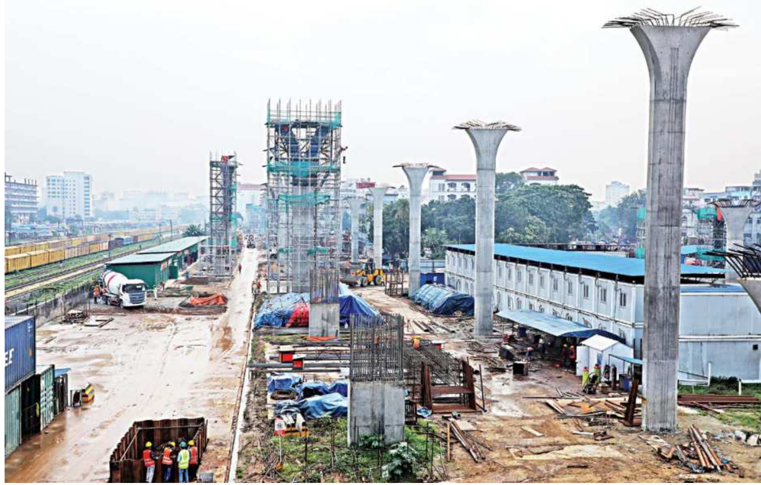
Construction work of Dhaka Elevated Expressway goes on in Tejgaon area yesterday. Road Transport and Bridges Minister Obaidul Quader last month said the whole project would be completed by June 2023. Once completed fully, the 19.73-kilometre expressway stretching from Hazrat Shahjalal International Airport to Kutubkhali on the Dhaka-Chattoogram highway is expected to help people get across Dhaka without facing the huge traffic congestion within the city.
