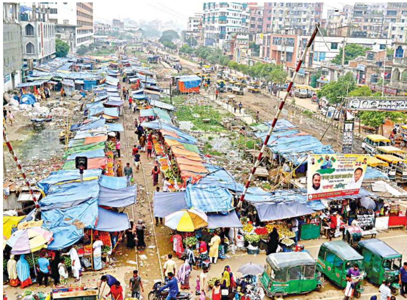
Temporary structures set up along the railway tracks poses a serious risk to both trains and passers-by. Even after repeated attempts, the authorities failed to evict such illegal structures that have sprouted beside the Dhaka-Narayanganj rail line. The photo was taken in the capital's Kamalapur-Jurain link.
