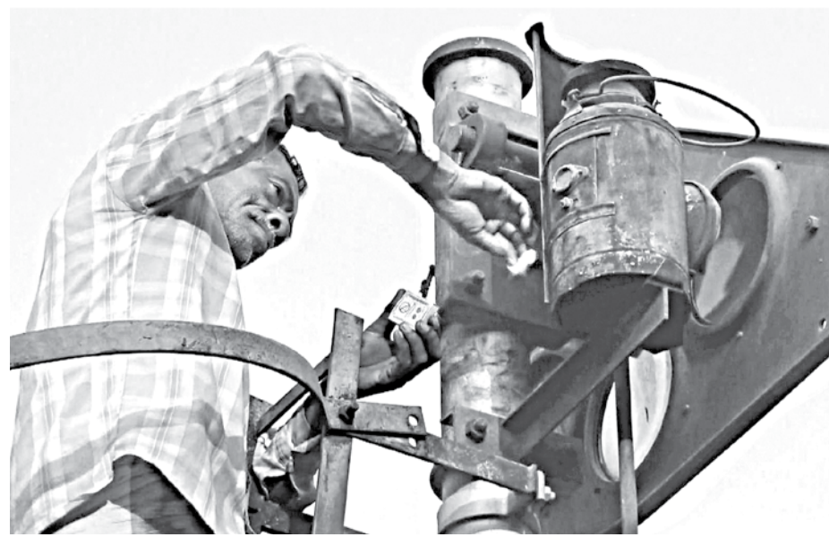
An operator lights up a kerosene-run lamp, which is part of a British-era signalling device installed at Mobarakganj railway station in Jhenidah's Kaliganj upazila.
