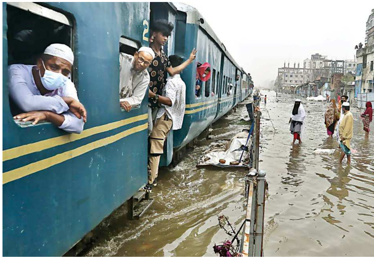
A train travels on rails that have gone under water after a not so heavy rain near Jurain Rail Gate area in the capital yesterday. Due to poor storm-water drainage, nearly a kilometre of the rail lines were under water.
