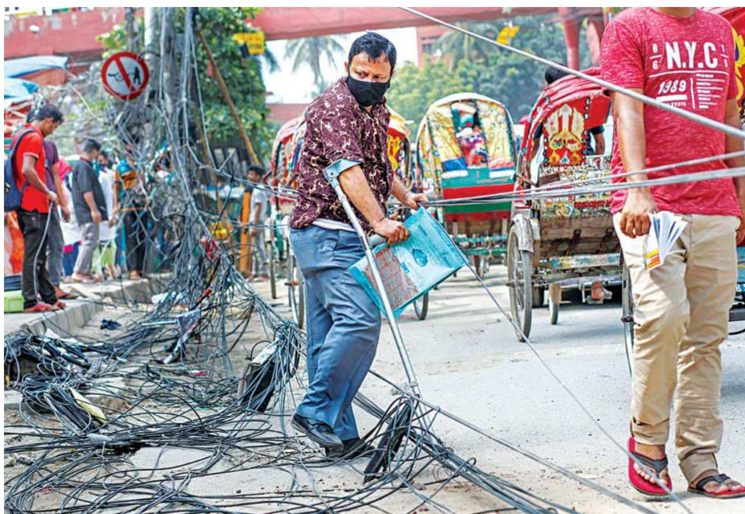
A man with challenges tries to cross the street avoiding the cables that have been left on the ground near Holy Cross Girls High School in the capital's Farmgate area yesterday. The authorities concerned cut the overhead cables but those were yet to be removed.
