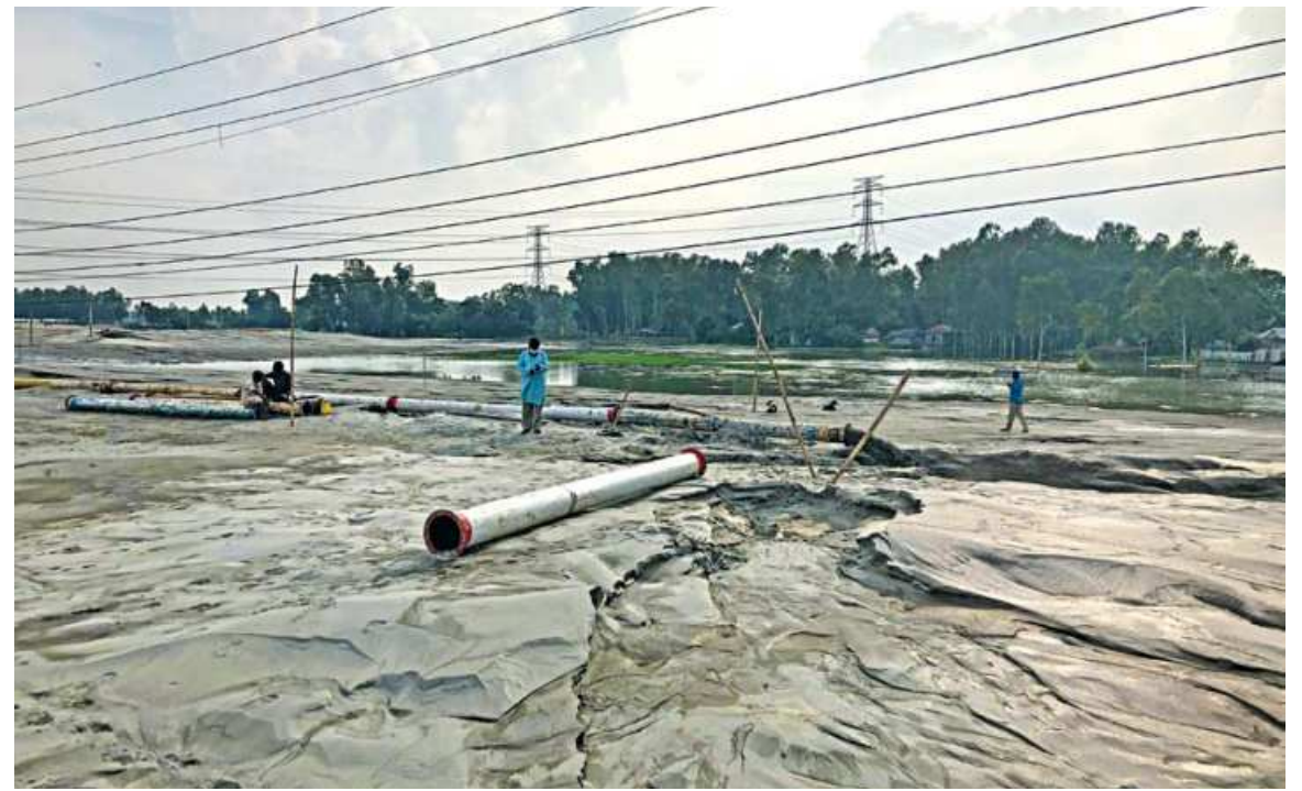
Earth-filling at the Sirajganj Economic Zone is underway. The country's largest private economic zone is expected to create five lakh jobs.
