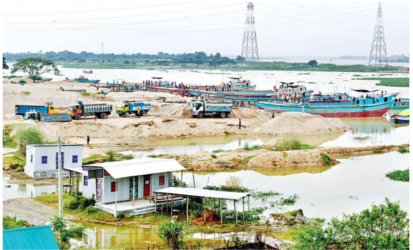
Encroachers have filled up significant portions of the Gumti river to run their sand trade right next to Meghna-Gumti bridge in Daudkandi, Cumilla. Similarly aggressive encroachment has caused the death of several rivers in the country.
