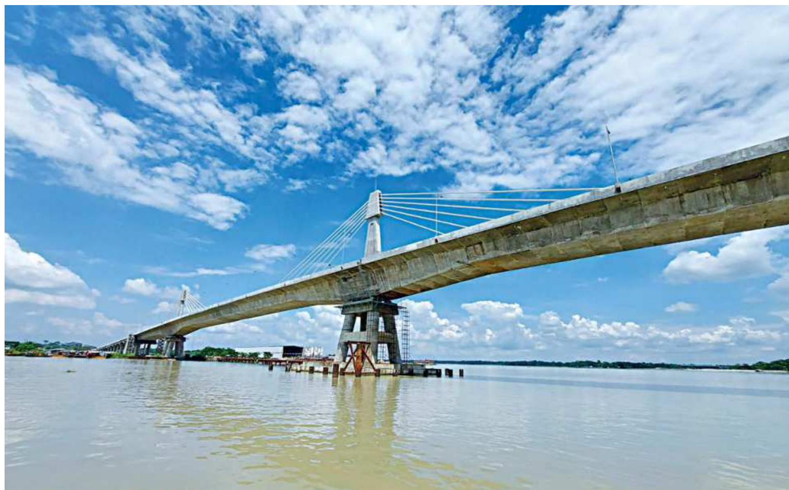
Payra bridge in Lebukhali area of Patuakhali district is scheduled to be inaugurated by Prime Minister Sheikh Hasina this month, according to project officials. The photo was taken last week.
