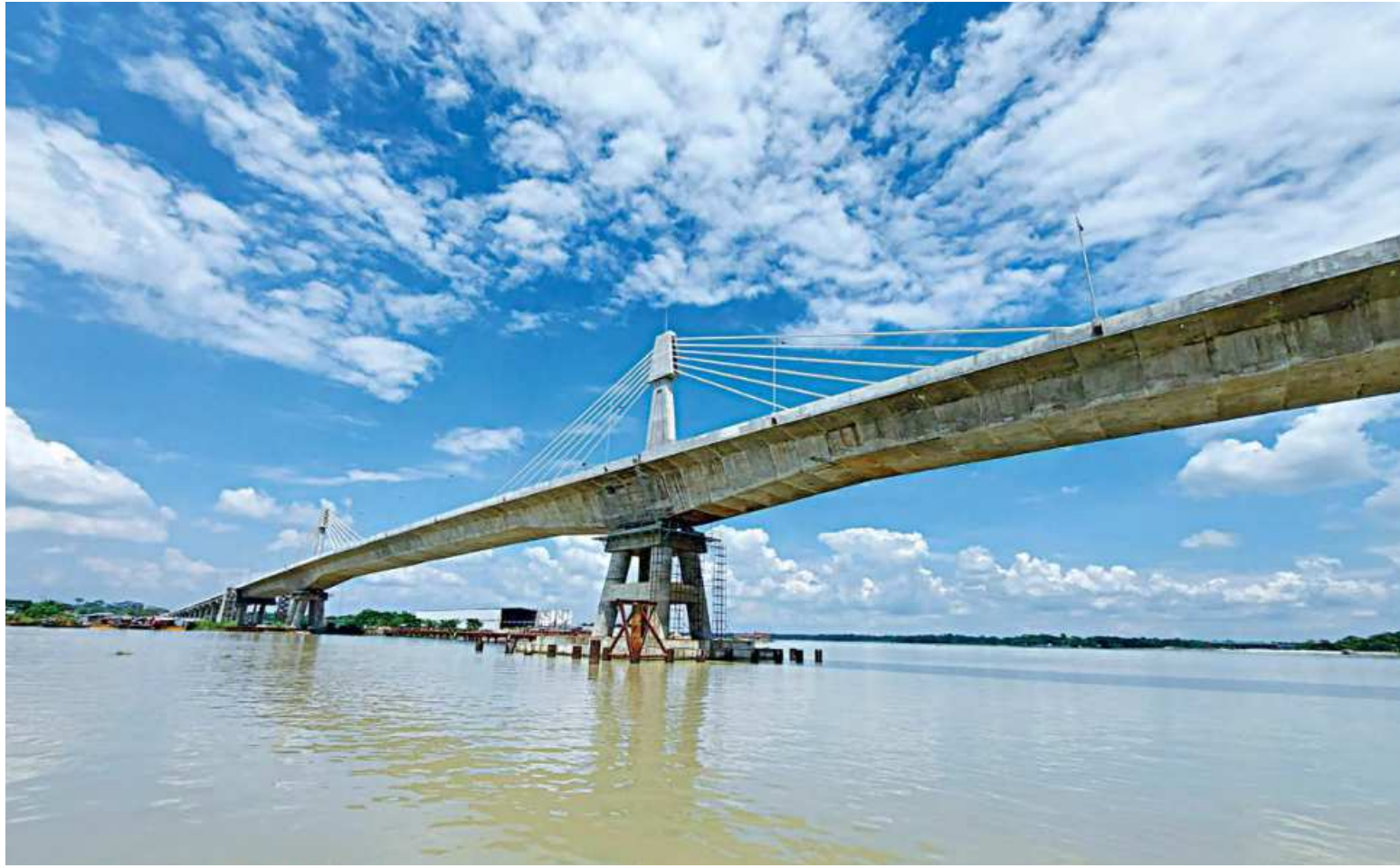
Payra bridge in Lebukhali area of Patuakhali district is scheduled to be inaugurated by Prime Minister Sheikh Hasina this month, according to project officials. The photo was taken last week.
