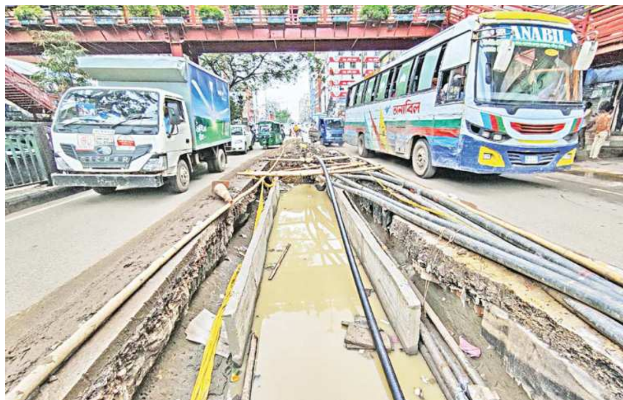
The DIC Road at the capital's Malibagh Chowdhury Para was dug right in the middle to install underground cables. A month on, the work is showing no signs of completion, piling an endless barrage of suffering on commuters. This photo was taken yesterday.
