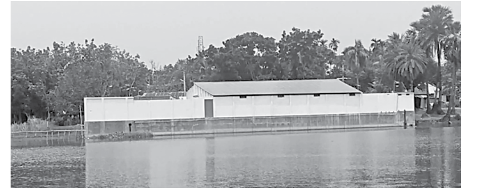
The oxygen refilling plant that was built encroaching on the bank of the Kaliganga river near Chheuria in Kushtia's Kumarkhali upazila.
