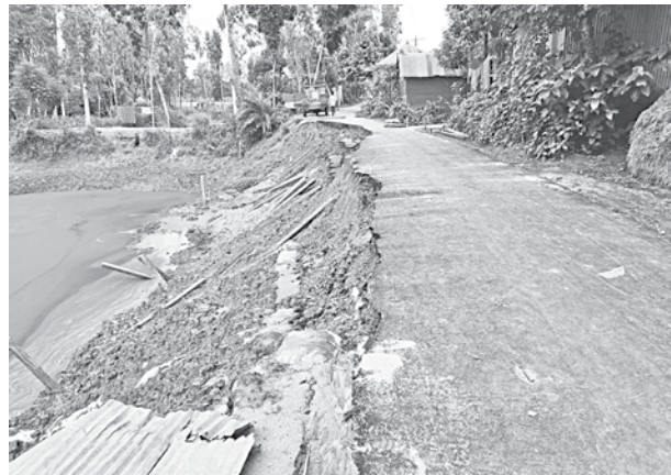
Portion of this newly built road at Ghargram village in Sirajganj's Tarash upazila collapsed in a roadside pond within 2 months of its construction.
