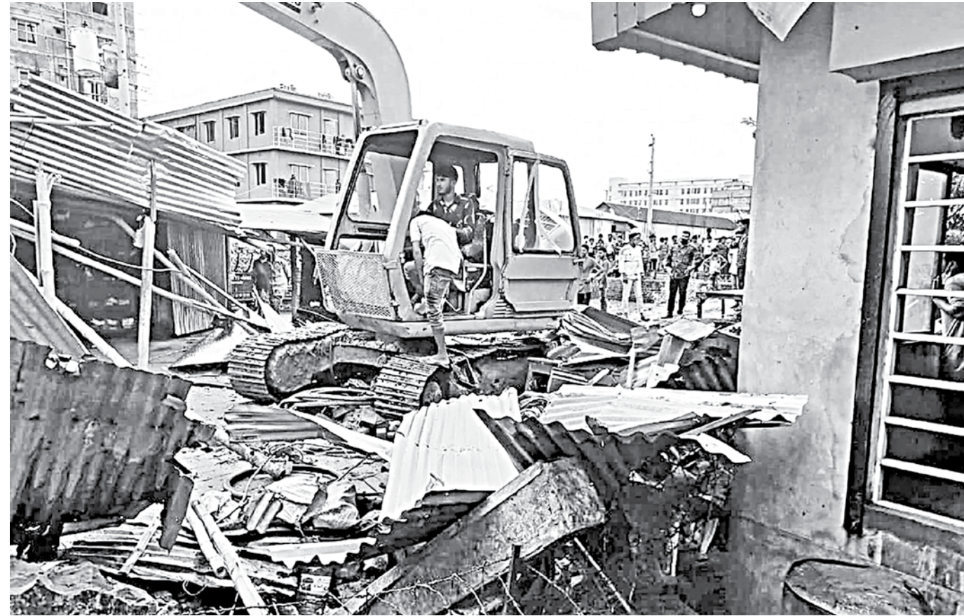
Blatantly disregarding law and court order, an excavator owned by the Gazipur City Corporation demolishes homes to make space for the city corporation's development projects. The photo was taken over a month ago.
