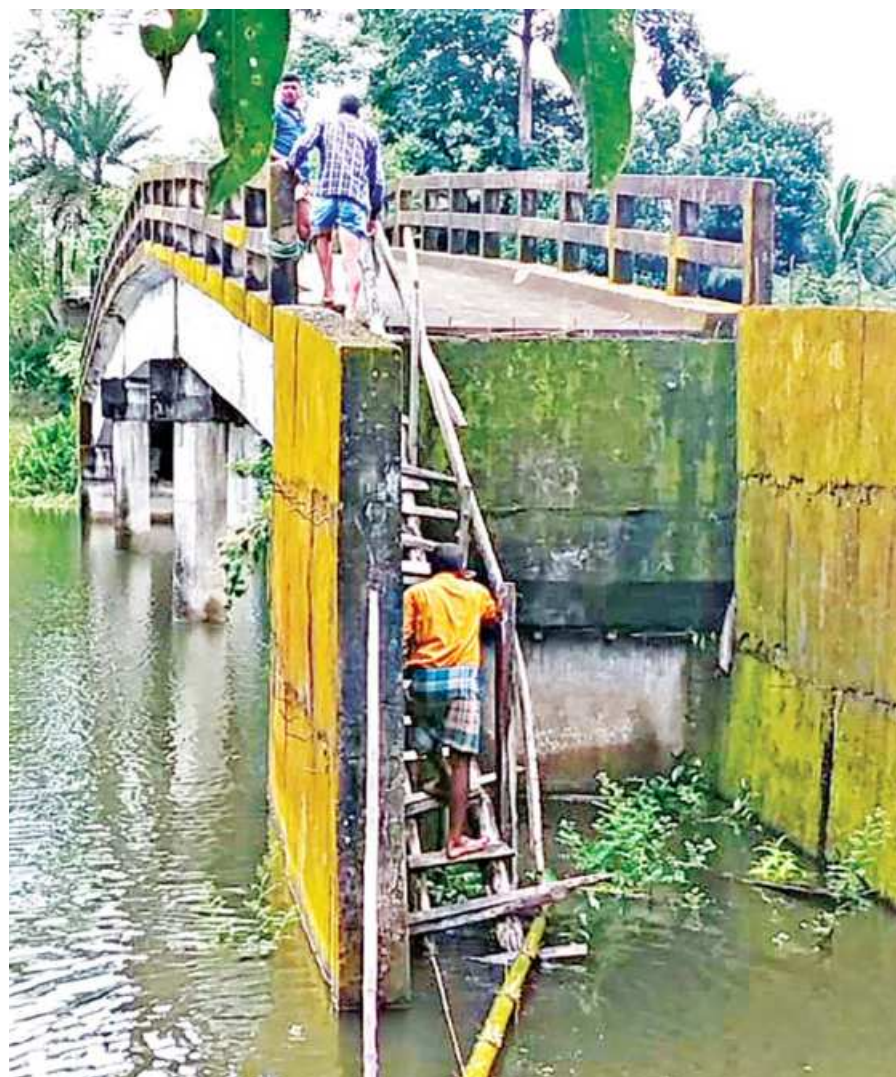
It is hard to believe that people have to use ladders like these to cross this bridge, built about 10 years ago over the Mainee river in Atarokchora of Rangamati's Longdu upazila. The contractor could not complete the construction work even after spending the total project budget of Tk 75 lakh. The photo was taken last week.
