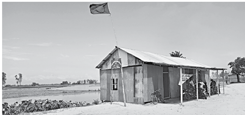
Teachers, guardians and locals voluntarily built this makeshift schoolhouse of Purba Satunama Aminpara Government Primary School on the right embankment of the Teesta river on September 11.
