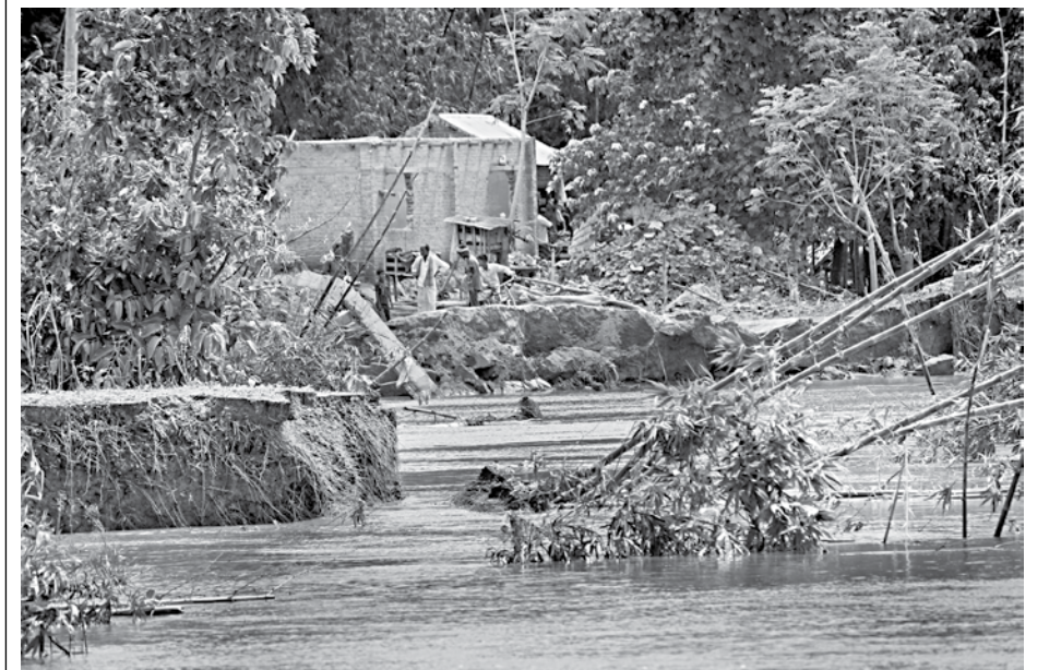
Over 100 families have been rendered homeless by the Padma river's erosion at Goadubi village under Sadar upazila of Chapainawabganj in last three weeks. PHOTO: RABTUL HASAN DOLLAR
