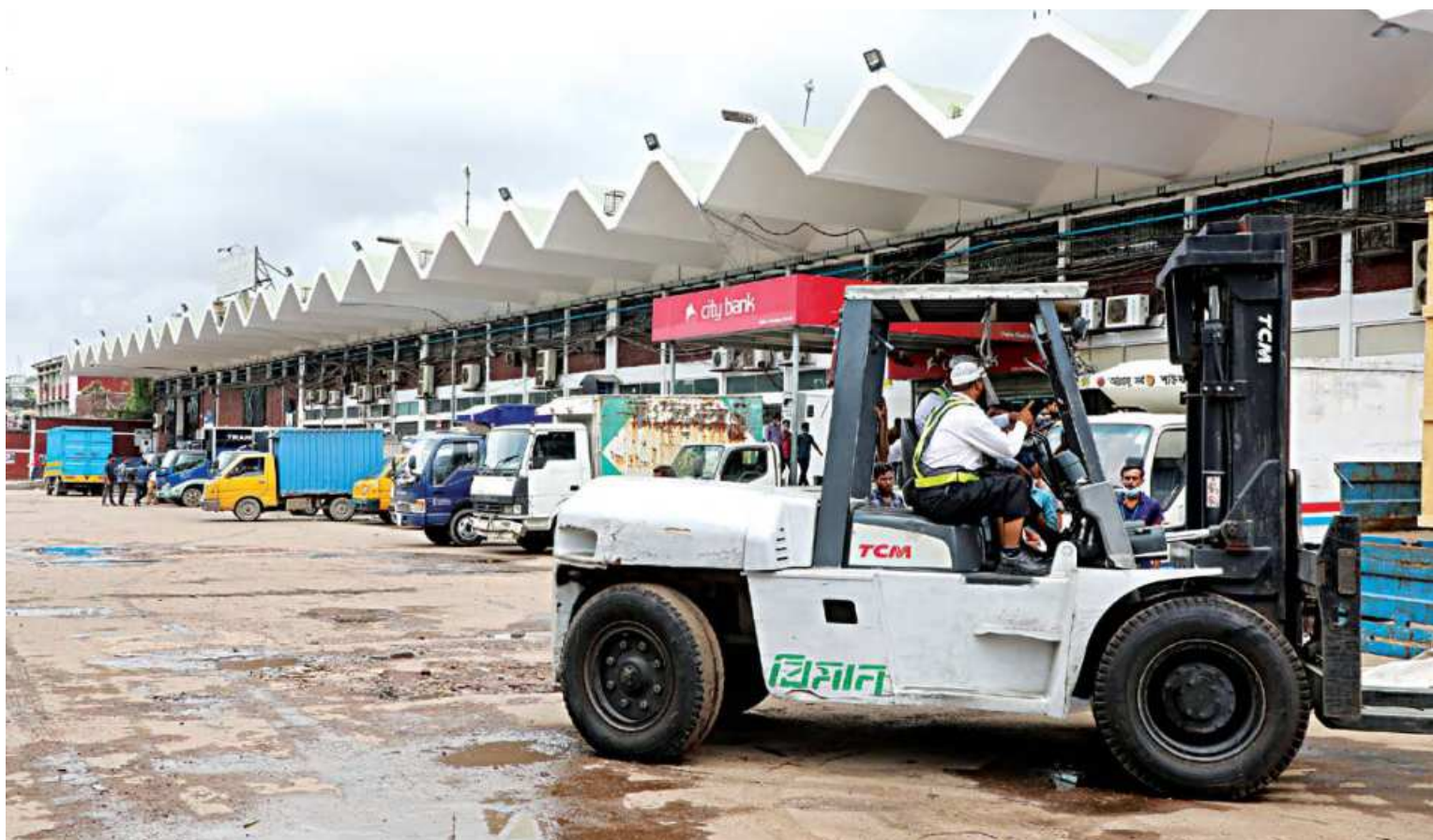
This cargo warehouse of Hazrat Shahjalal International Airport in Dhaka has become overloaded amid allegations that exporters treat it as their own personal space, storing goods without any bookings. The photo was taken yesterday. PRABIR DAS
