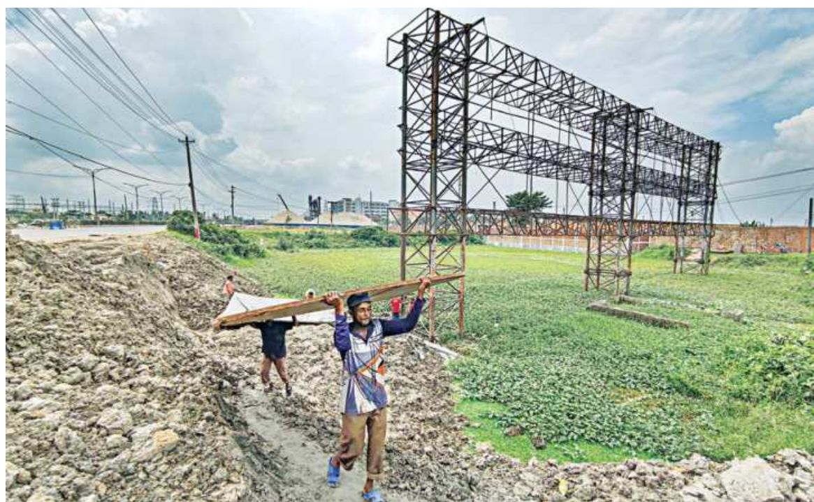
Workers dismantling a large hoarding from the side of the Dhaka-Aricha highway near Amin Bazar to make room for a new bridge there. After a bridge subsided disrupting traffic flow on the key highway, the authorities have decided to build the new structure with better capacity.
