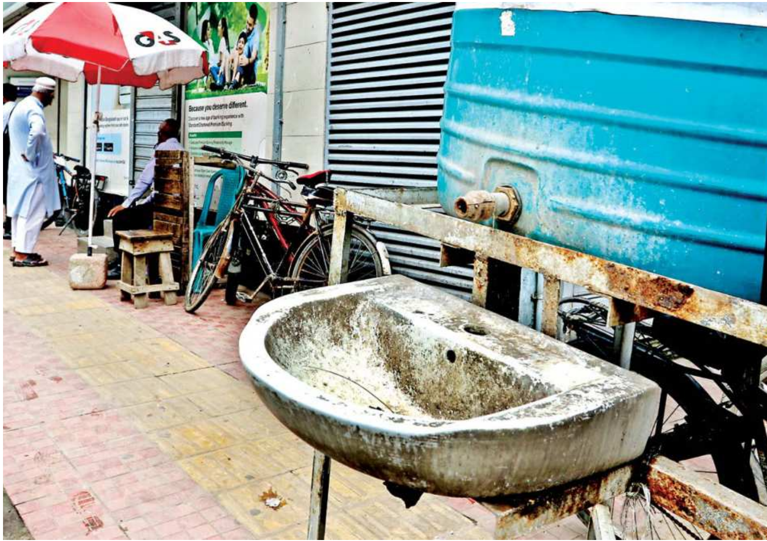
To help the capital's residents resist the coronavirus, Dhaka Wasa took an initiative of placing several hand washing facilities across various locations of the city. Only that most of them are lying out of order, with no water in the tanks and even the taps missing. This photo was taken yesterday from Kazi Nazrul Islam Avenue near Karwan Bazar.
