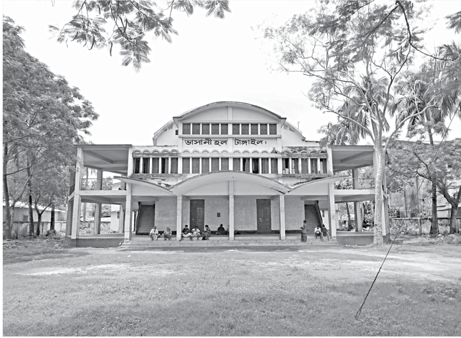
The Bhasani Hall in Tangail, the epicentre for entertainment and cultural activities of the town, has remained abandoned for the last three years due to its dilapidated condition.
