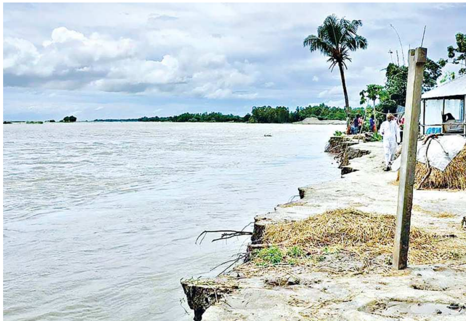
Around 20 homes have been devoured by the Padma at Aria-Gohailbari of Pabna Sadar upazila over the last two months. Villagers alleged that encroachers have been lifting sand and soil from the area, resulting in the river erosion. The photo was captured a few days ago.
