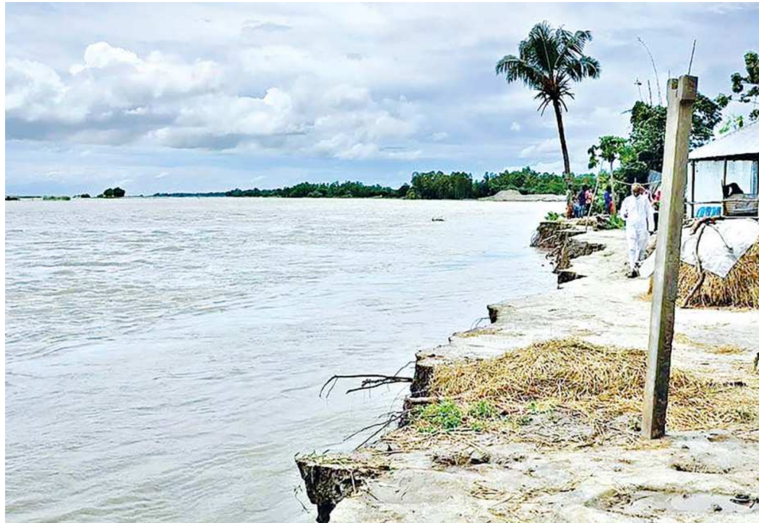
Around 20 homes have been devoured by the Padma at Aria-Gohailbari of Pabna Sadar upazila over the last two months. Villagers alleged that encroachers have been lifting sand and soil from the area, resulting in the river erosion. The photo was captured a few days ago.
