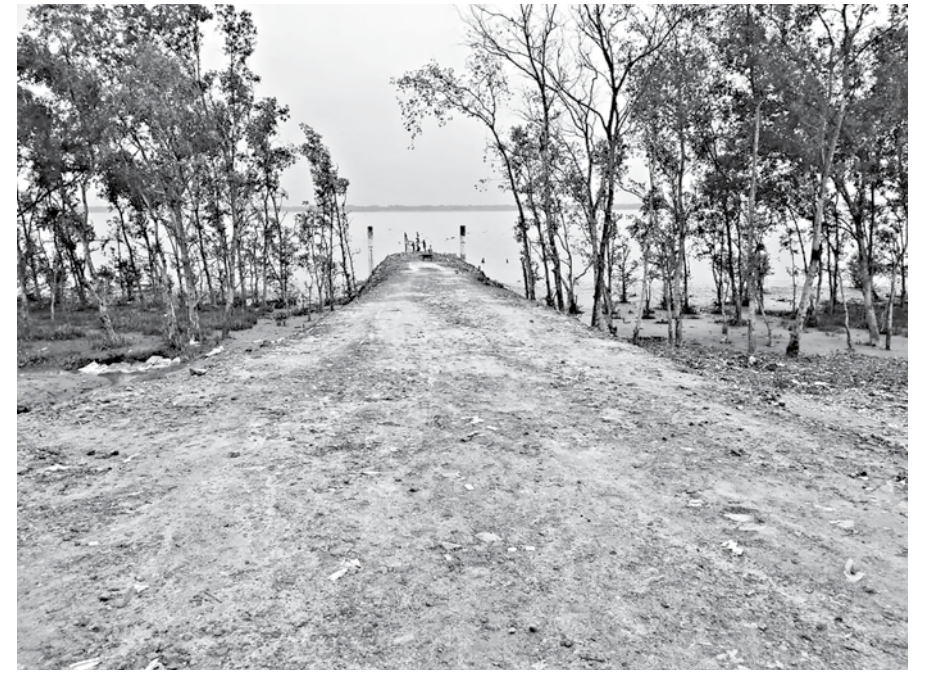
The under-construction ramp of the Rayenda ferry terminal on the bank of the Baleshwar river in Sharankhola upazila of Bagerhat. PHOTO: COLLECTED
