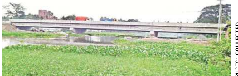
The bridge, constructed with poor clearance in Jashore's Jhikargachha bazaar area, makes it impossible for medium-size vessels to pass.
