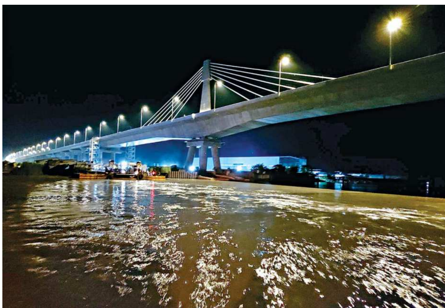
The Payra Bridge on the Barishal-Kuakata highway was lit up on an experimental basis on Saturday night before the inauguration of the much-awaited bridge. The authorities plan to open the cable-stayed bridge to public soon.
