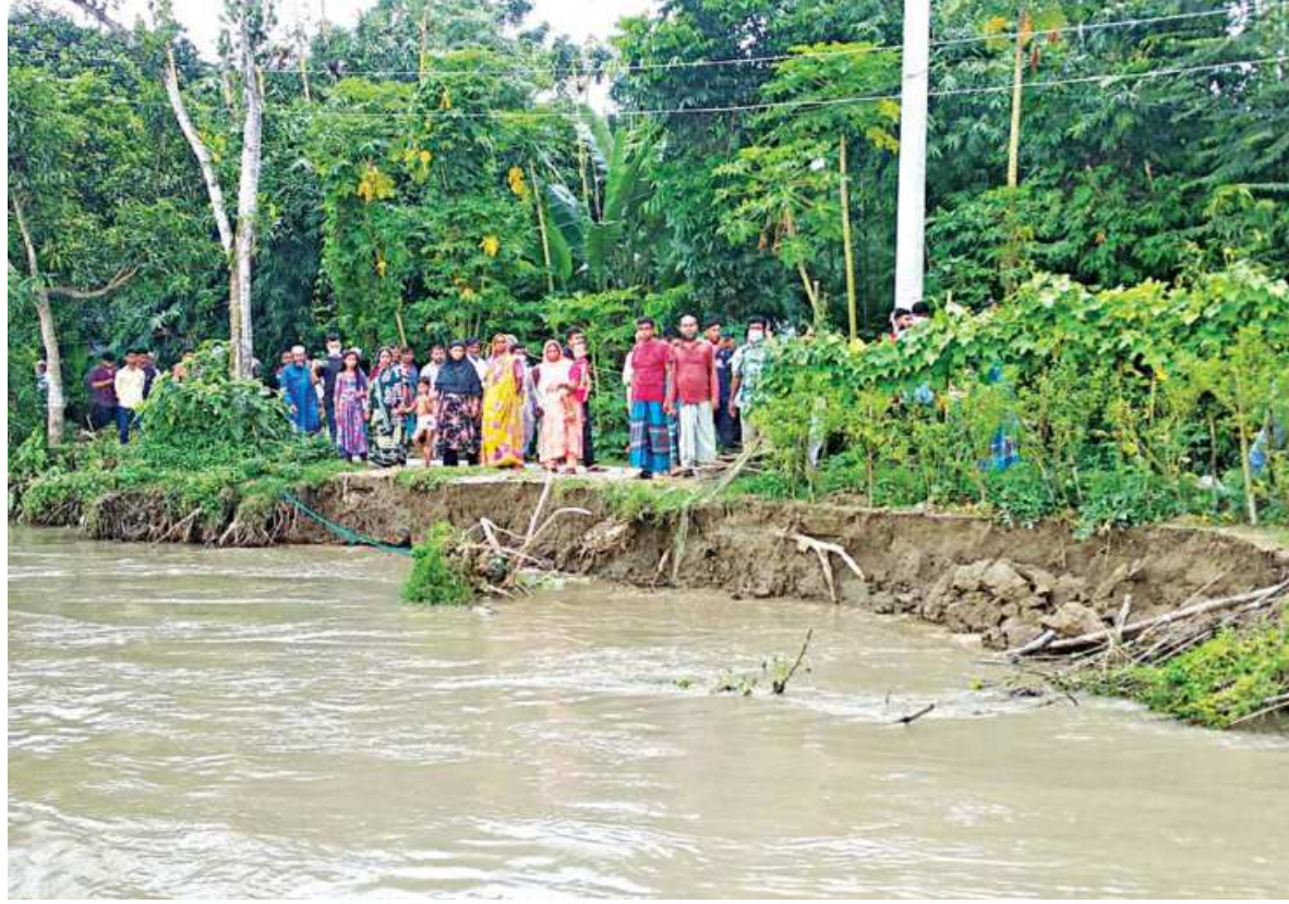
Concerned locals gather near the Silimpur-Karatia embankment, popularly known as Tangail town protection embankment, as erosion of the Pungli river caused multiple cracks in it. They requested the authorities to take necessary measures immediately to reduce damage. The photo was taken yesterday.
