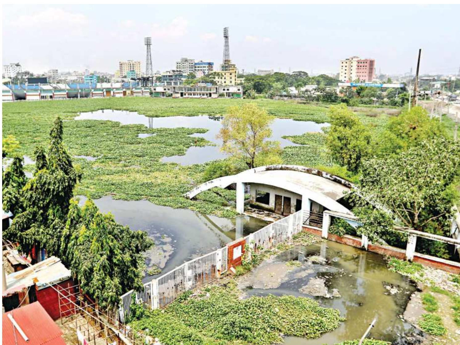
A large field just outside the Khan Saheb Osman Ali Stadium in Narayanganj's Fatullah has been under water for several months as there is no drainage system in place. The stadium cannot be used for months every year due to this perennial waterlogging problem. The photo was taken yesterday.
