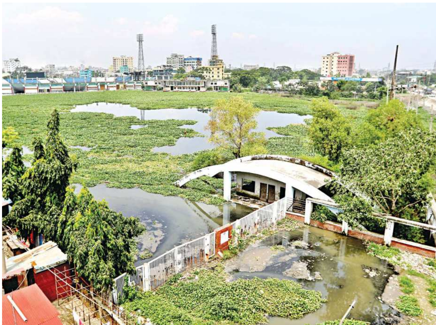
A large field just outside the Khan Saheb Osman Ali Stadium in Narayanganj's Fatullah has been under water for several months as there is no drainage system in place. The stadium cannot be used for months every year due to this perennial waterlogging problem. The photo was taken yesterday.
