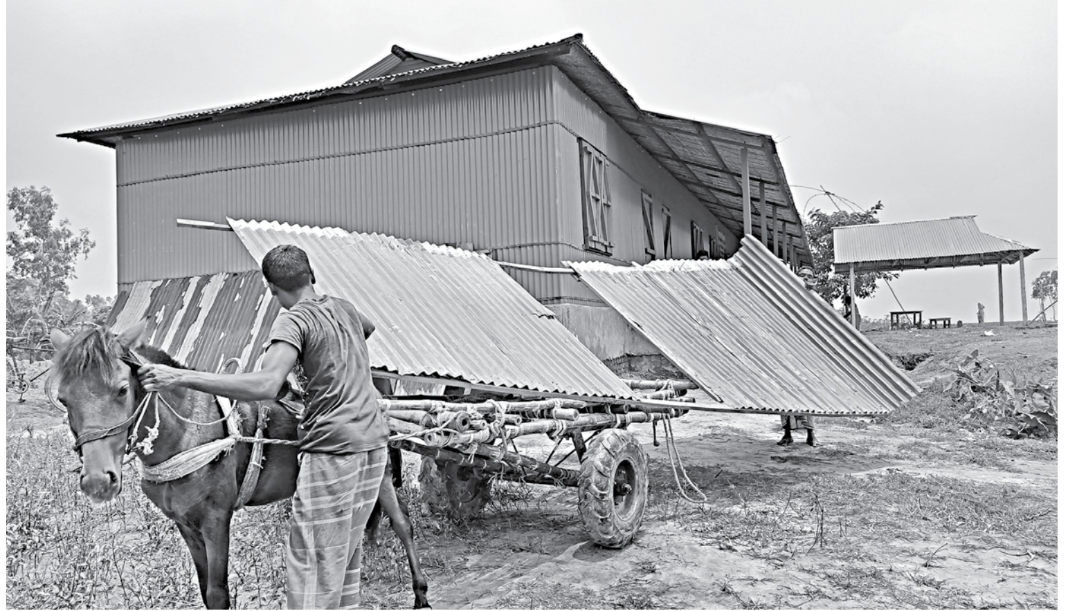
The movables of Pashchim Bajra Government Primary School in Ulipur upazila of Kurigram are being removed before a furious Teesta devoured its building.
