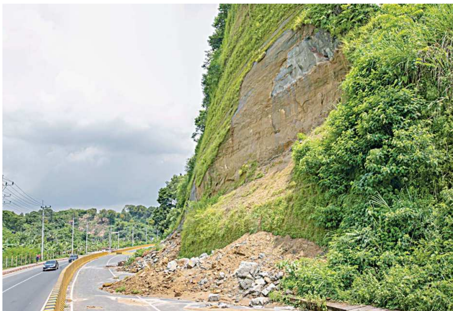
This dual-carriageway, connecting Foudjarhat and Bayezid in Chattogram, was built cutting part of a hill. A large chunk of earth recently fell on the road and the authorities, deeming it unsafe, have closed off one side of the road at Jangal-Salimpur and set up contraflow on the other side. The photo was taken yesterday.
