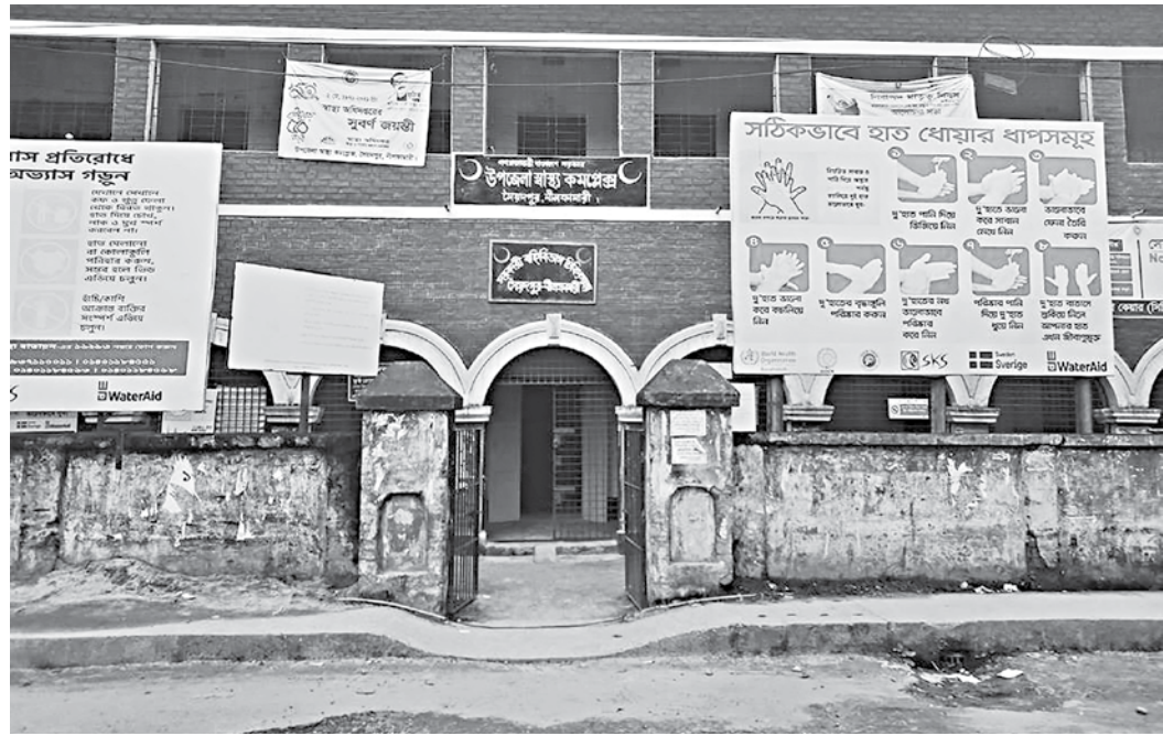
The upazila health complex in Saidpur town of Nilphamari.
